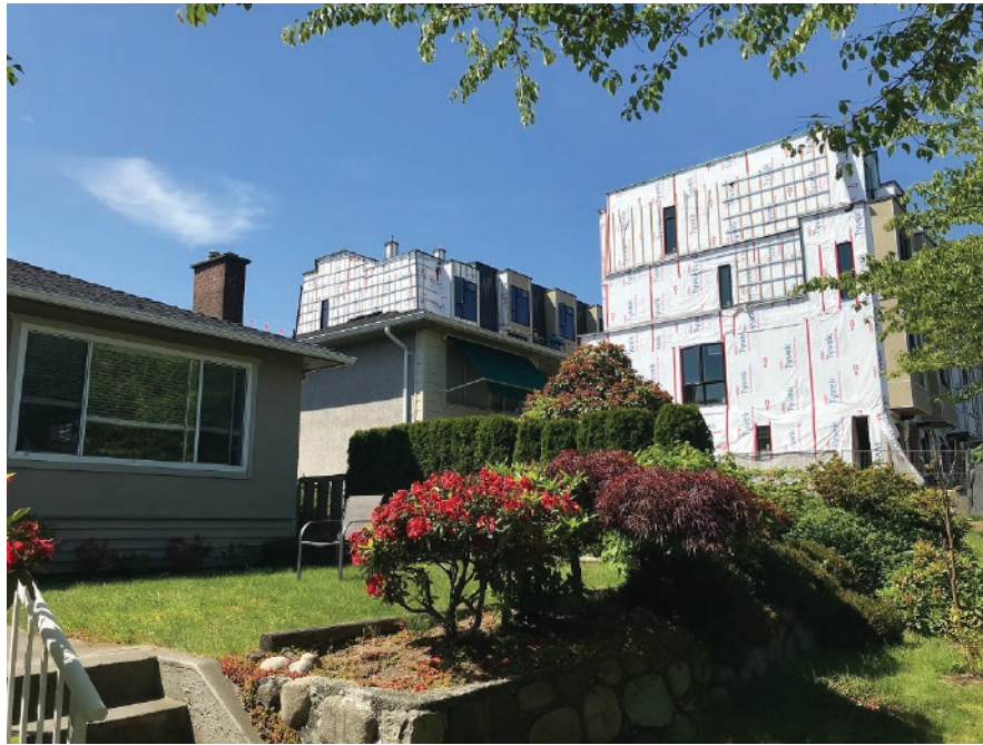
Figure 14. New Buildings Next to Old
